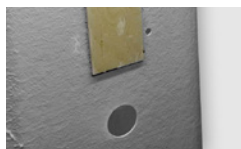
Additional Backing & Drilling
