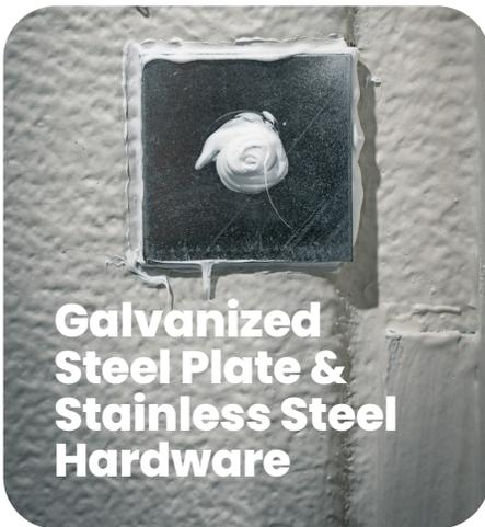
All safety bars are supported on the back of the unit with a galvanvanized steel plate which is then siliconed to avoid steam or water penetration.
